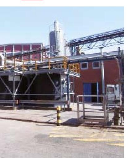
Top left: Complete structure made from GRP profiles
